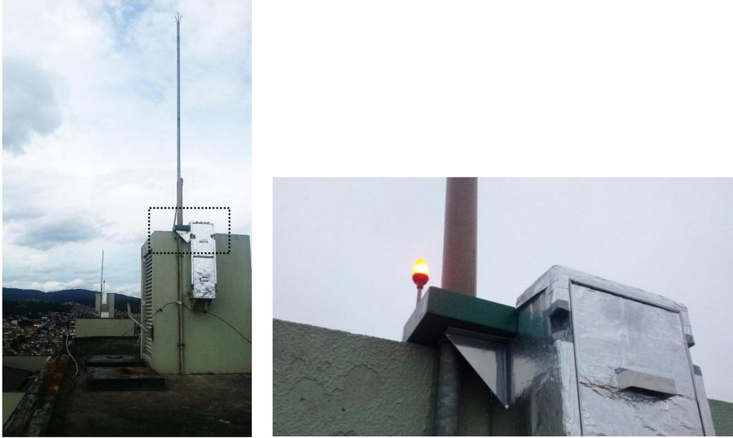
Figure 5. Current sensor installed on the lightning rods (left) and detail of the installation (right).
